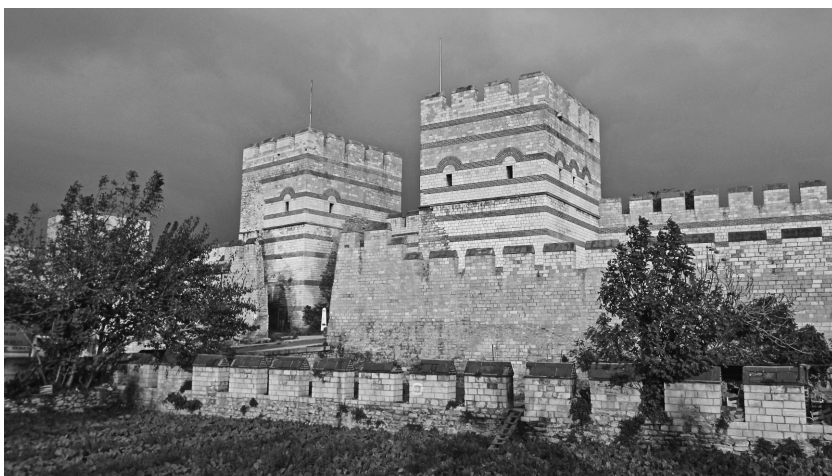
Figure 14 An extensively restored section of the Theodosian Walls, showing the three lines of defense; the moat or ditch before the first line has been filled in.
